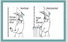
in the direction shown and keep panels plumb. Secure panels to studs with drywall screws. Drive screws until panel is tight against framing and screw is just below board surface without breaking the
