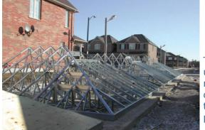
The roof truss system used for the garage roofs was assembled on the ground and then lifted up into position.
