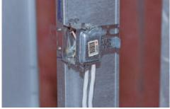
Steel framing is pre-punched for electrical wiring. Heating and ventilating ducts, plumbing and drain pipes can readily be installed.
