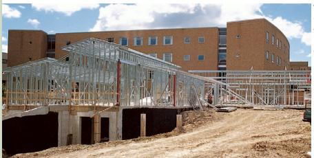
"Light steel framing was used to retain the ratings, yet be used in a residential framed manner."
