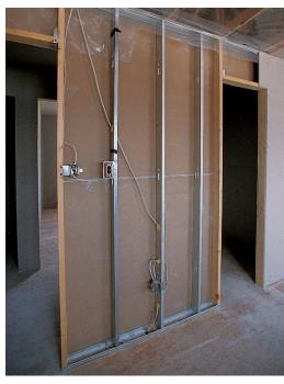
The main benefits to light steel framing are cost savings from no call-backs for warpage, nail-popping or cracks, plus ease of use.
