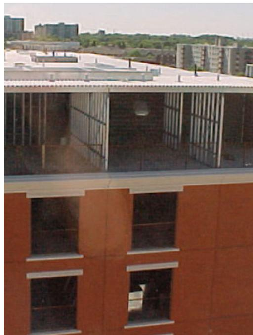
standpoint is the floor system. " Actually John Wilkinson came up with the idea on an earlier condominium project. It worked so well we used it here too. We wanted to reduce impact sound floor-to-floor, and he got the idea from the approach used in commercial buildings. The result is a composite floor where concrete is poured onto a corrugated steel deck with depths ranging from 89 mm to 152 mm (3-1/2" to 6") and no joists for a total floor depth of
