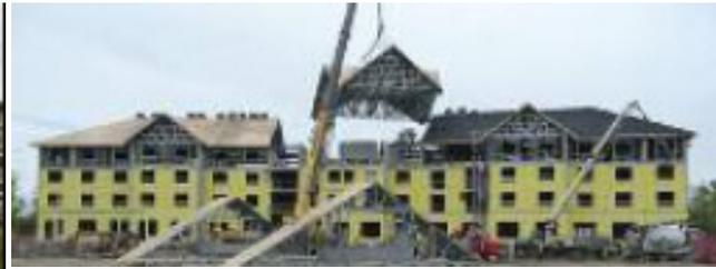
"Light steel framing is cost effective, produces a straight wall and provides excellent sound ratings. For this project, it provided flexibility and met our design needs."
