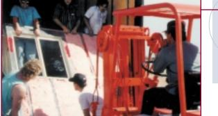
Mexico (Photo: Armour Steel Framing) Workers unload pre-assembled panels for model homes in Tijuana, Mexico.
