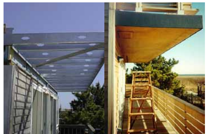
Figure 9 - New Jersey Site Under Construction
