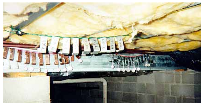
Figure 5 - Stud specimens in Leonardtown Site crawlspace. Note the uncoated C-sections in the background show red rust after just two months of exposure.
