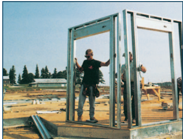
Steel stud walls can be stick-built or panelized
