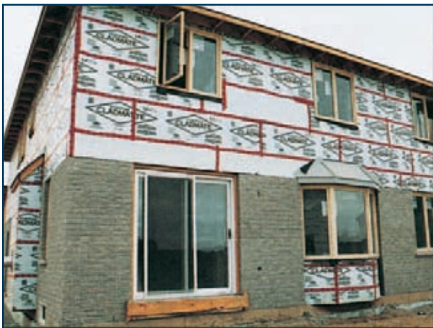
Insulating rigid sheathing is an important part of the building envelope.
