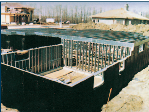
Basements can also be framed out of steel.
