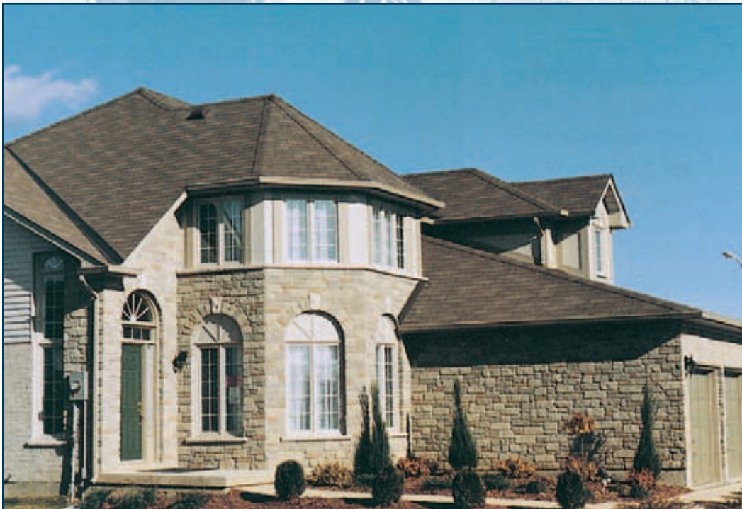
The first Homesteel project was built in Ancaster, Ontario. This home featured steel wall studs and floor joists in an otherwise traditional home.
