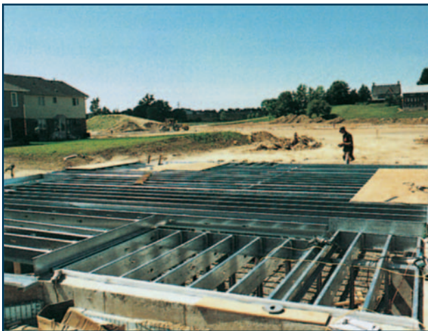
Steel floor joists are easily installed and can span continuously across supports.
