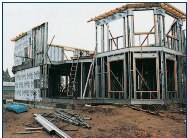
The Ancaster Homesteel Project utilized stick-built construction methods.
