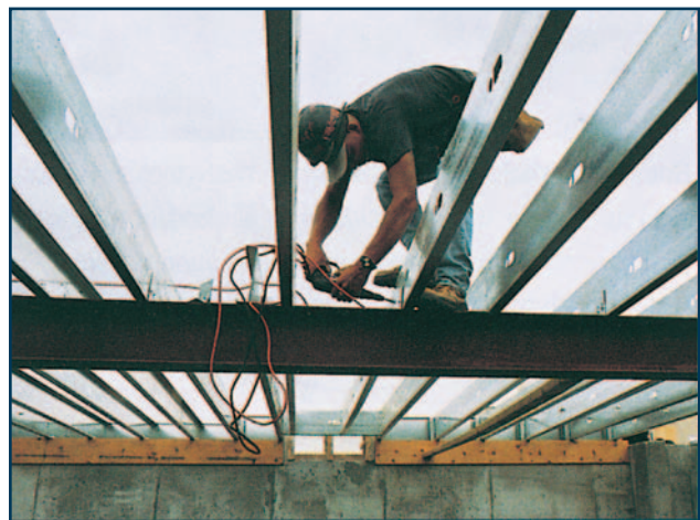
Screwing is the most common means of connecting steel framing
