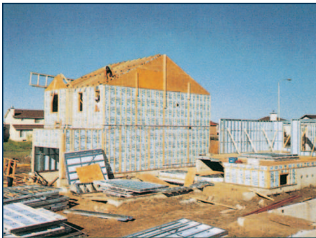
This project in Ottawa was built up from prefabricated panel assemblies.
