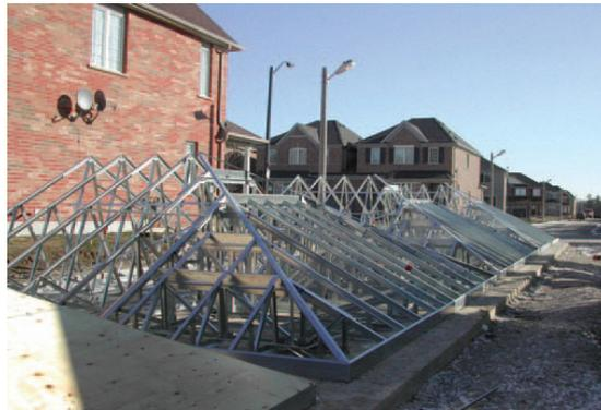
The roof truss system used for the garage roofs was assembled on the ground and then lifted up into position.
