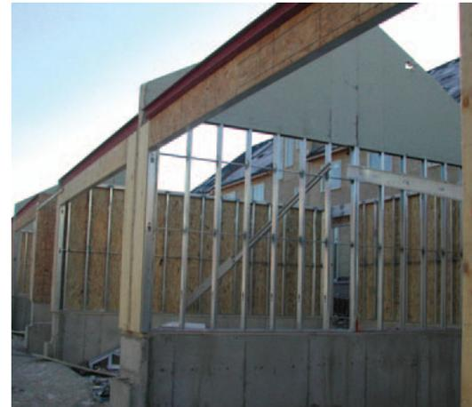
Genesis™ pre-engineered and pre-assembled panels were used to frame both the townhomes and the garages.
