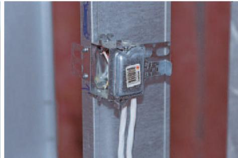
Steel framing is pre-punched for electrical wiring. Heating and ventilating ducts, plumbing and drain pipes can readily be installed.
