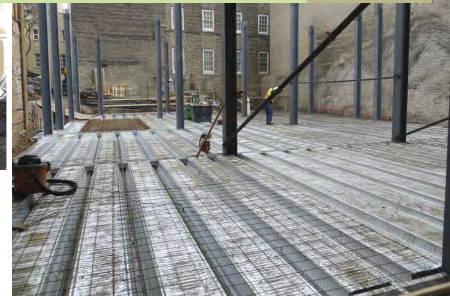
ComSlab at ground floor, ready for concrete.
