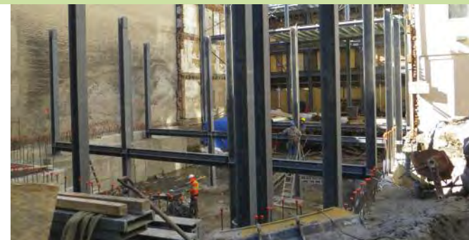
Construction of new structural steel and ComSlab.
