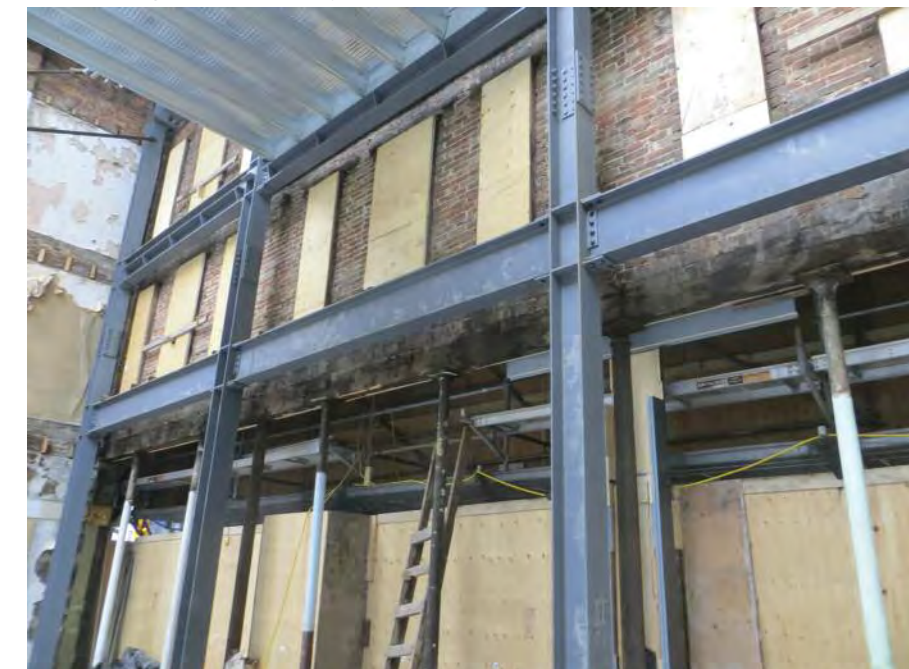
ComSlab at ground floor, ready for concrete.
