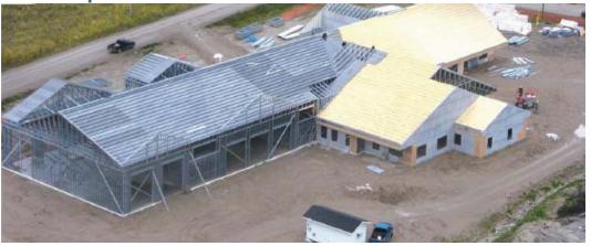
It was a race against time to build the facility to a closed-in state in one construction season – including the pouring of a 2,323m<sup>2</sup> (25,000 sq. ft.) engineered concrete slab. As well, fabrication and erection needed to be as simple as possible given the lack of a local highly-skilled labour force.
