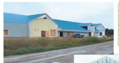
Precut material and components, were assembled over the course of the winter months in Moose Factory. Construction on site started in the spring. Wall panels were shipped to the site in July and assembly of the superstructure took place in July and August.
