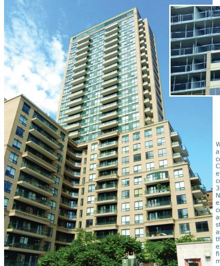
When you're building a 32-storey high-rise condominium in one of Canada's largest cities, every bit of space counts. For Toronto's 349-unit Bloor Street Neighbourhood, the exterior envelope consists of preassembled light steel framed panel assemblies to which the attractive Dryvit exterior, in a Terraneo finish, are fastened mechanically.
