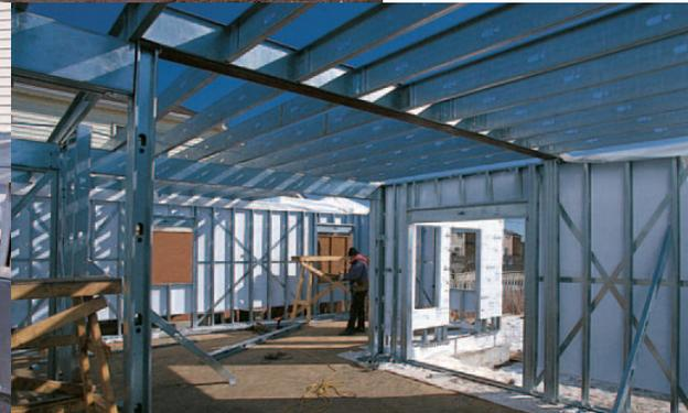
Light steel framing won't rot, shrink, swell, split, or warp, is not affected by insects and, of course, does not add fuel to a fire. As well, steel's high strength-to-weight advantage means that it can span greater distances and thus provide greater design flexibility with larger open spaces minus intermediate columns or loadbearing walls.
