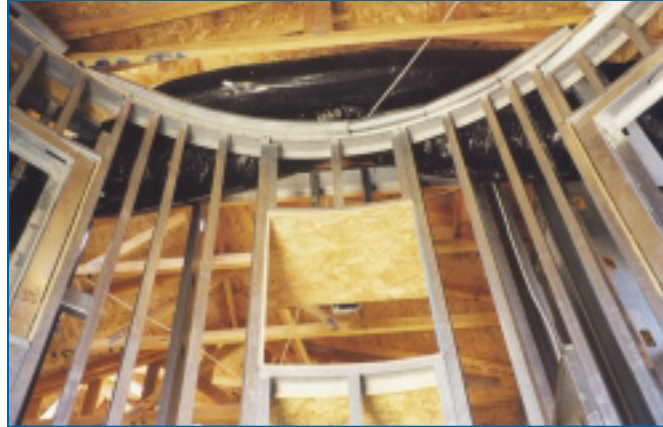
The flanges and web in non-loadbearing track can be cut to allow for quick and simple fabrication of a curved wall.
