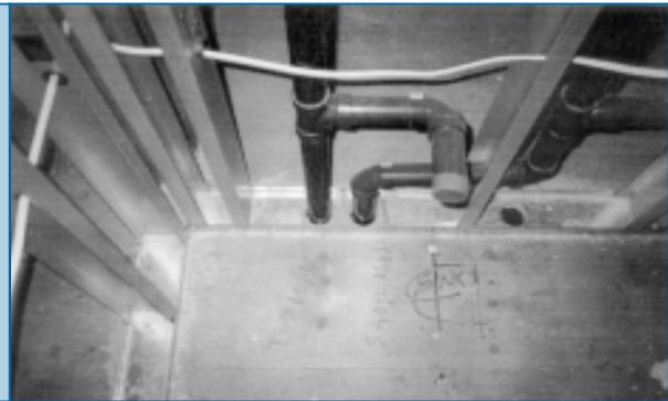
Aligned knockout holes in these floor joists allows straight through passage of electrical and plumbing (water pipe) services. Grommet protection for the services is installed in the knockouts.
