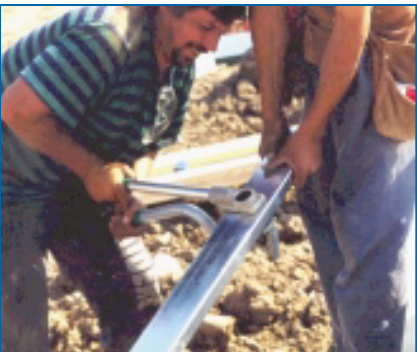
A manual hole punch can be used to create holes in non-loadbearing LSF.
