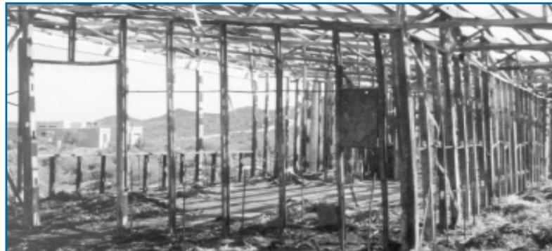
Photo 2: "Steel framing still standing after the fire."
