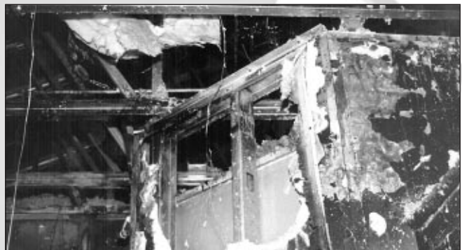
Charred steel studs from 1996 Brentwood, CA home fire maintained structural integrity.
